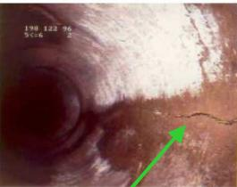
**BABCA 03** Longitudinal fracture at 3 o'clock
