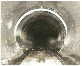
**BAJ B** Displaced pipes
